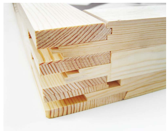
Shorted tenons allow stormproofing of sashes without breakout.
